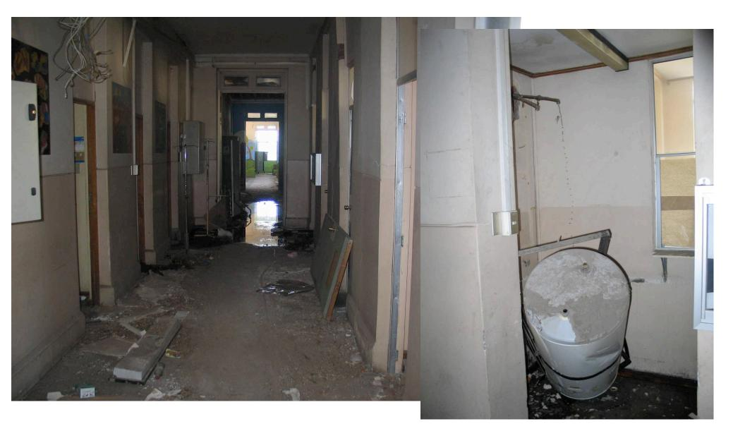
Continuing water damage at Talca Hospital. Water is leaking from water heater on right. Building was closed due to nonstructural damage, dominated by water.
