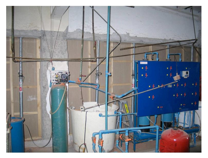
2005 building; Los Angeles Hospital. Infill masonry wall collapses on to distilled water equipment, spilling two 150 gallon containers; water leaks past perimeter edge of slab to OR suite below, closing 3 or 6 ORs
